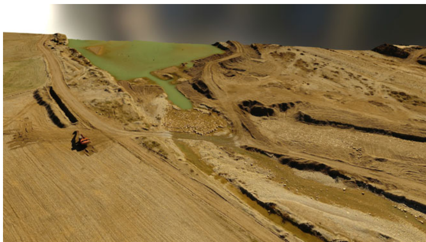
FIGURE 4. A 20m wide Assyrian dam across the Chai Bastora river, commissioned as part of canal building by the Assyrian King Sennacherib (early 7th century BCE). It is under threat by gravel mining and seasonal flooding. 3D model based on drone imagery © Directorate of Antiquities of Erbil/Khalil Barzinji, 23 January 2017. Results of the Erbil Plain Archaeological Survey (EPAS) led by Jason Ur, see their original model on Sketchfab .
